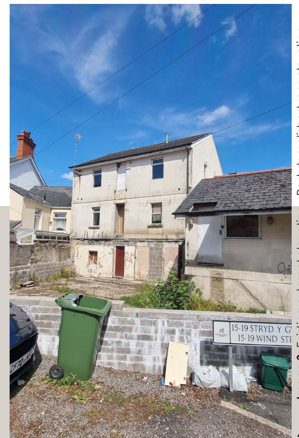
Image 3: Existing external elevation - Part demolished rear elevation
