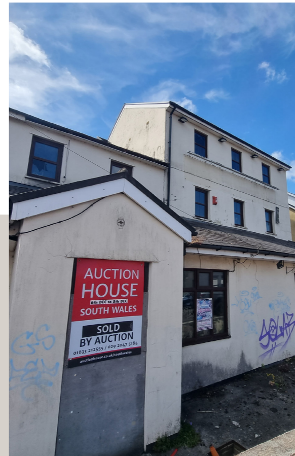
Image 2: Existing external elevation - from junction (Front Elevation)
